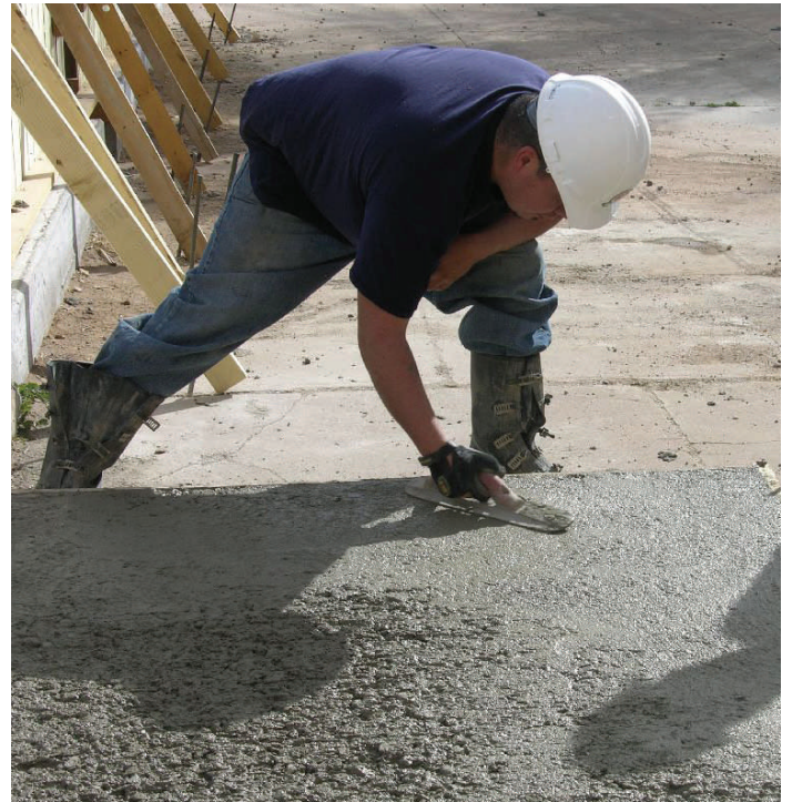
LCC Building Technology students Anthony Martinez, Ralph Gallegos and Peter Olivas start laying concrete slab on a teaching module at the LCC Building Trades Facility. (Photo at right) Building technology student Nathaniel Montoya starts the finishing process on a slab at a teaching module. For more information on building technology, call Joseph Montoya at 505/454-2586.
