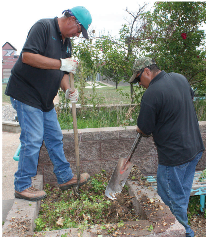
Desiderio Sena and Leon Roybal work outside the Student Services Building recently. Physical plant workers continue to work on Luna Community College's landscaping plan.
