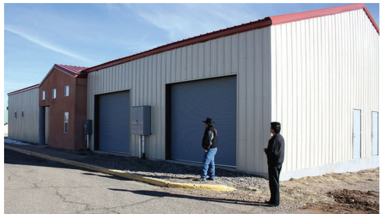
Luna Community College President Dr. Pete Campos and LCC Facilities Director Ron Gonzales evaluate both the inside and outside of the unfinished Collision Repair Building. The college hopes to secure resources to finish the building.
