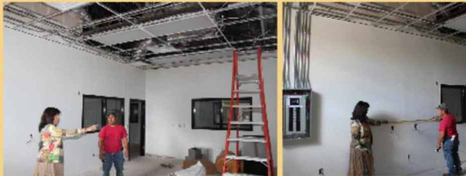
Cross Connection Contractor Foreman Mark Sanchez, Title V Director Lorraine Martinez go over measurements in the Electrical Lab.
