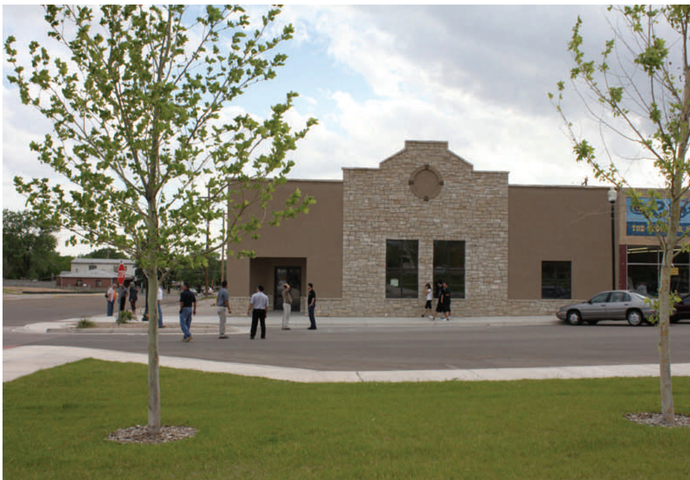
Luna Community College Board of Trustee members, along with LCC President Dr. Pete Campos and guests take a tour of the nearly-completed exterior renovation of the LCC Regional Health and Safety Center in Santa Rosa.
