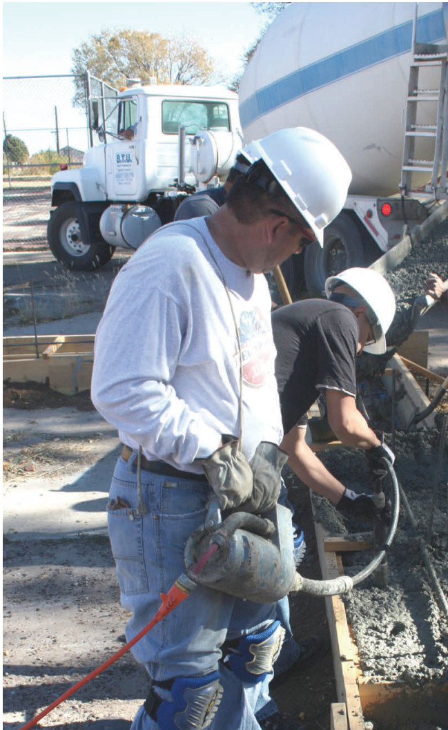
Luna Community College building technology students on Friday received first-hand experience on how to do a foundation pour. The students, along with instructor Joseph Montoya, worked on a foundation for a new teaching module building that will be built by students next to the trades department. Pictured clockwise are: Montoya and Kevin Gutierrez; Anthony Martinez and Peter Olivas; Ralph Gallegos, Gutierrez and Montoya; Isaiah Dominguez, Montoya, Joseph Quintana and Gallegos; Dominguez and Quintana; Gallegos and Montoya. .
