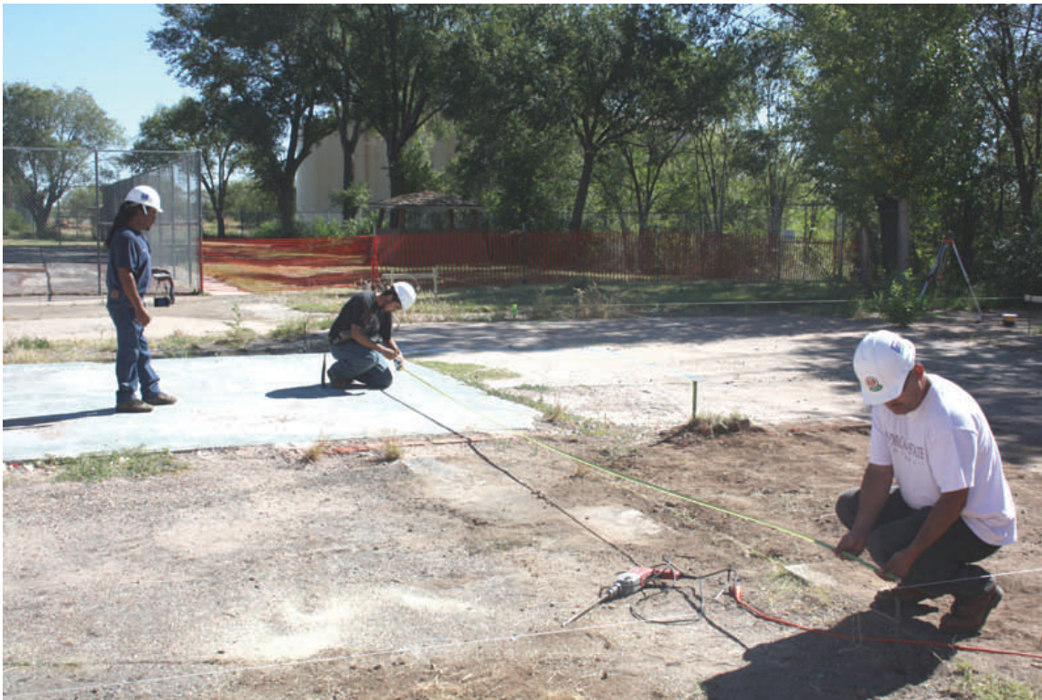
Luna Community College students Ralph Gallegos (right) and Joseph Quintana began site layout procedures for new teaching module home to be built at the Trades Department. Instructor Joseph Montoya is teaching students correct procedures for this type of work.
