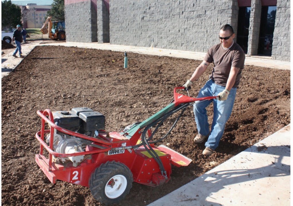
Luna Community College Physical Plant employee Juan Macias works on renovation project outside the administration building. Doing more work from within and not outsourcing as much is part of LCC's cost-cutting measures.
