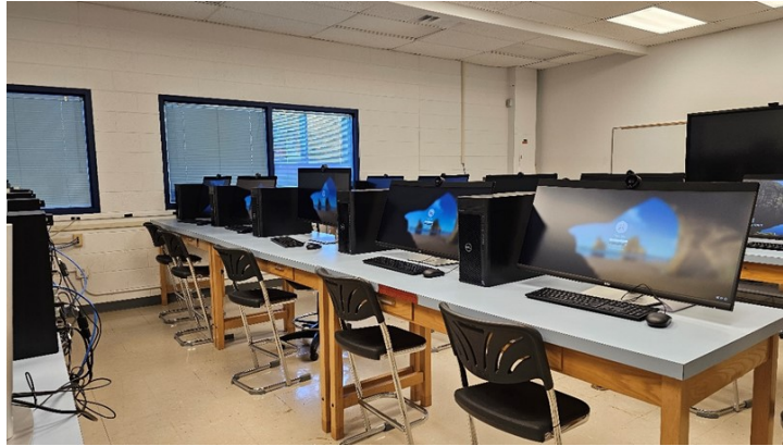
The Luna IT department has been installing new hardware throughout campus.
